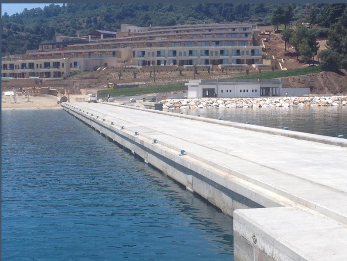
Bridge' s final shape
