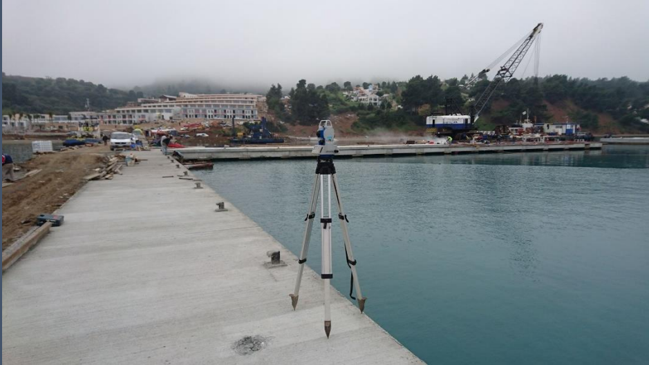
Intermediate phases of works, surveying
