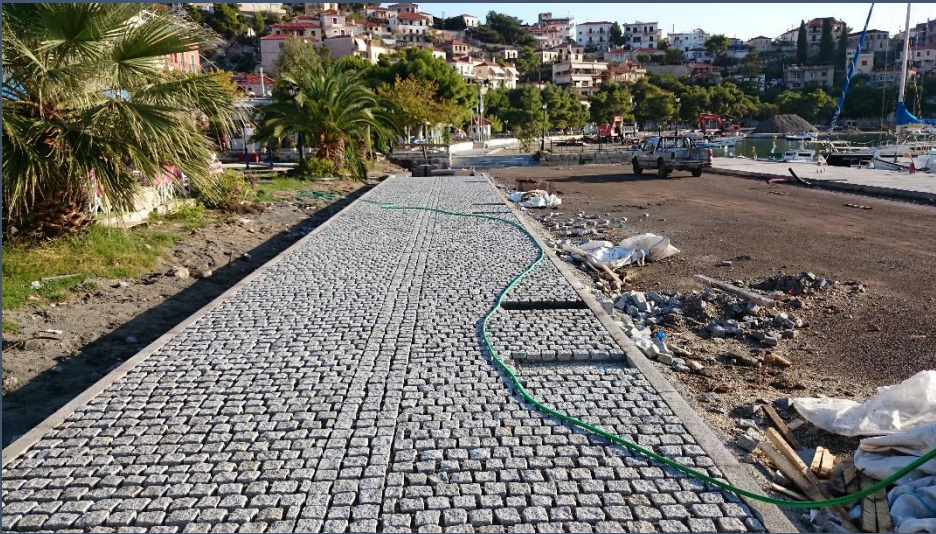
Traditional stone-laying pavement
