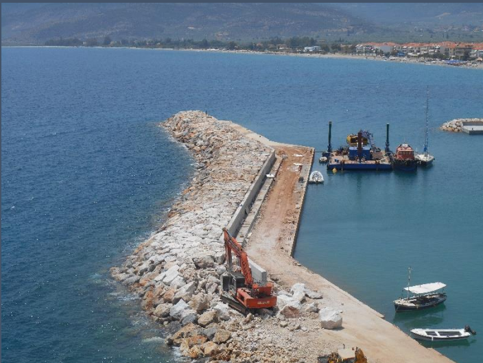
Windward pier under construction
