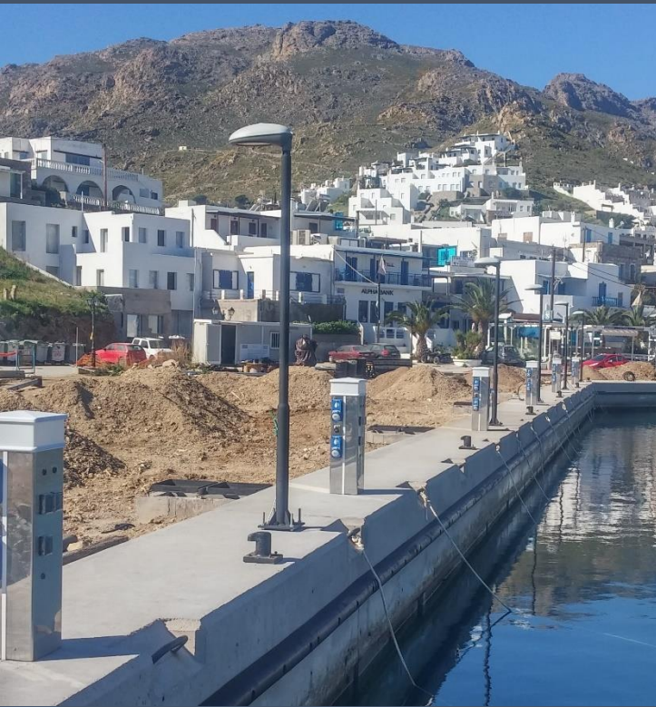
View of the dock with the pillars
