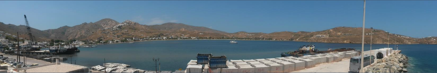
Concrete blocks construction on land
