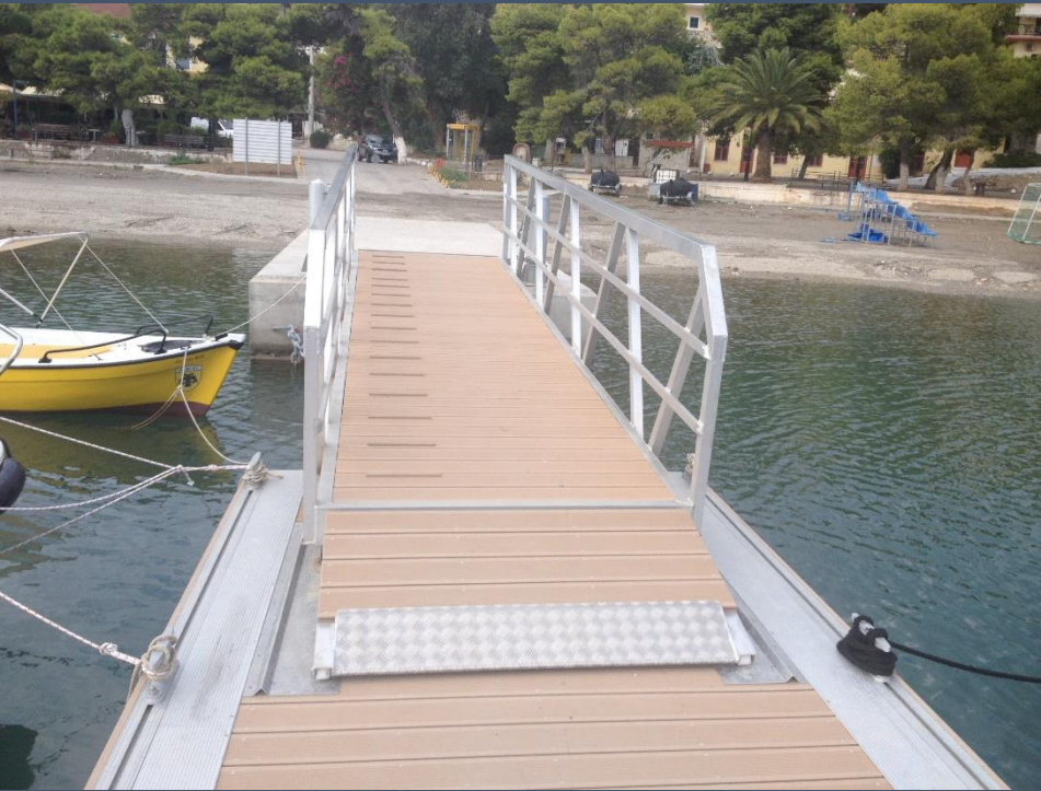
Floating pontoon' s connection bridge.
