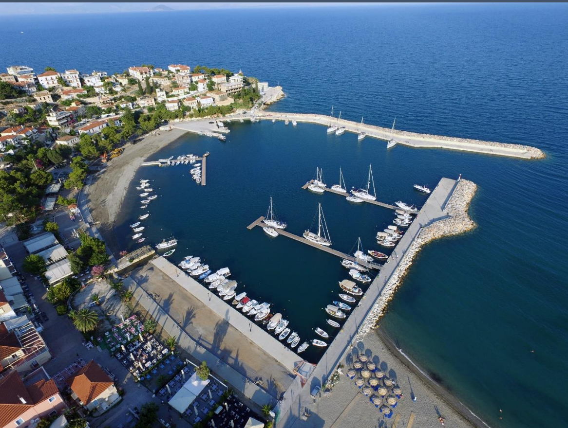
Drone view, May 2015
