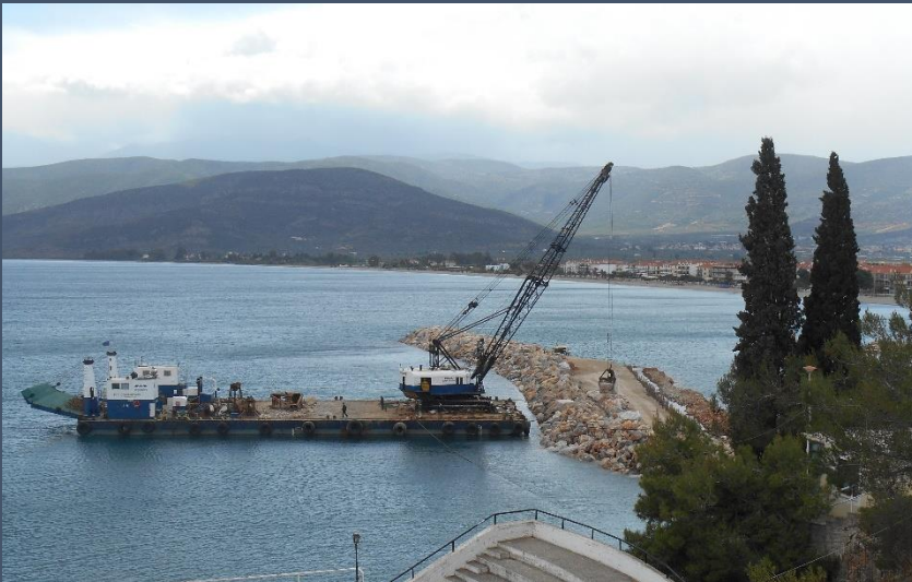
Concrete block placing by the floating crane
