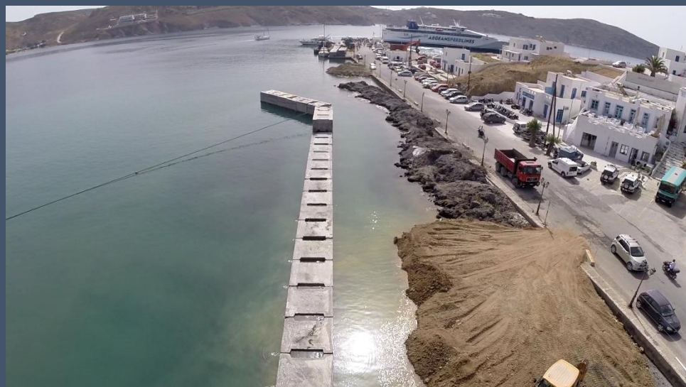
Concrete blocks placed in the sea
