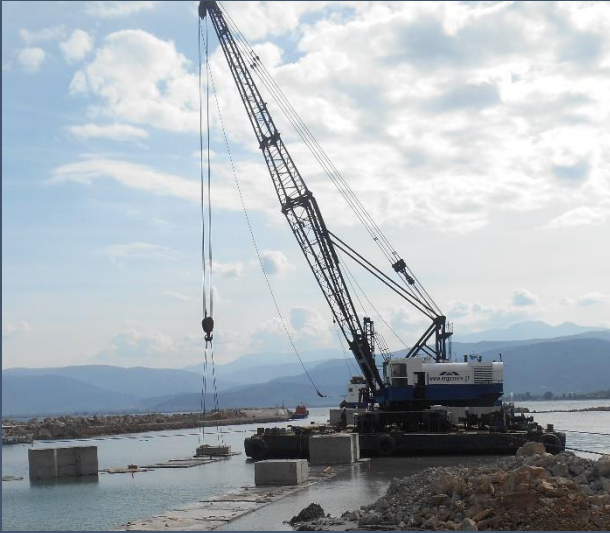
Concrete block placing by the floating crane
