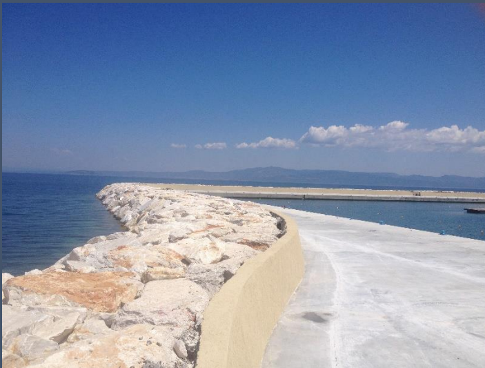
Breakwater protection by big stones, brought on site by boat
