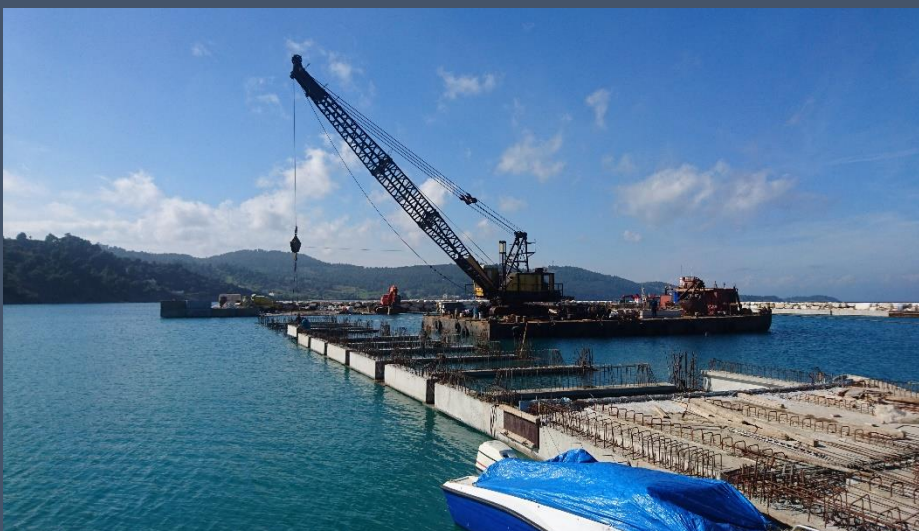
Bridge precast parts mounting
