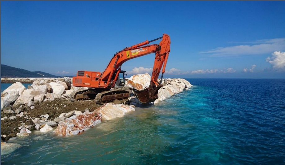
Breakwater stones placement by excavator
