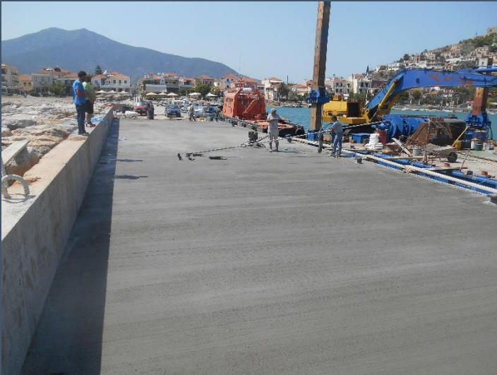
Concrete pavement finishing
