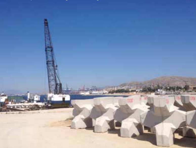
Accropode moulding and loading in Piraeus - 2017
